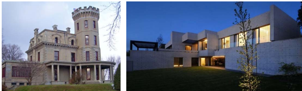
Figure 15. Recognizing Concrete for Use in Architecture 1876 and 2010 [98, 8]
